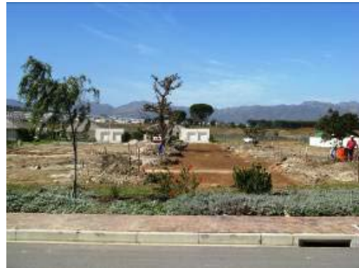
Phase 2A services complete – waiting for the road
