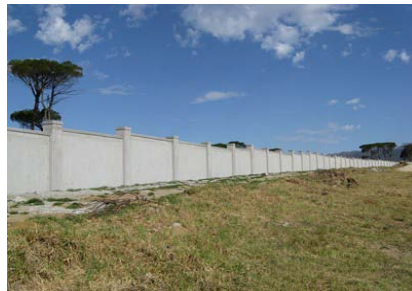
North/east boundary wall in phase 2
