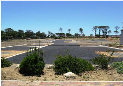
Phase 3A services for the Garden Cottages
